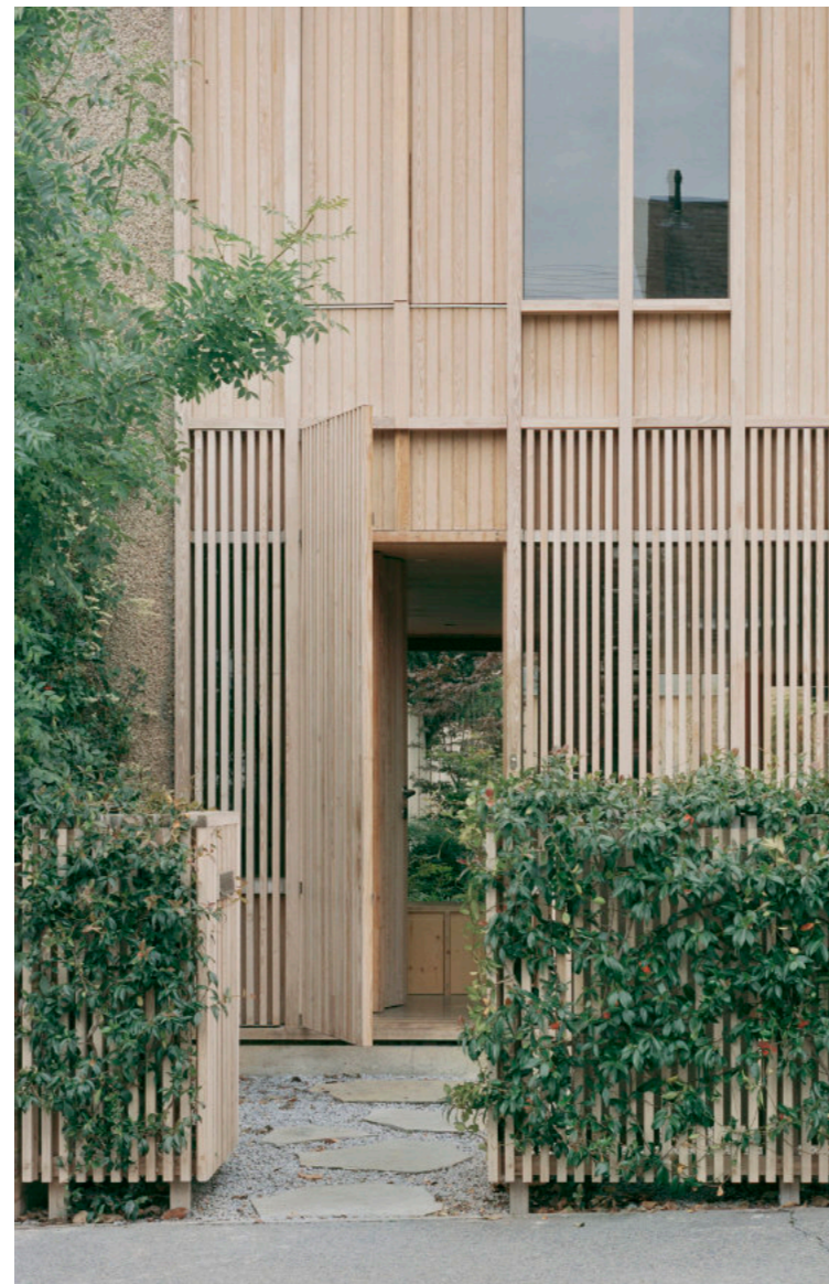
The Spruce House, ao-ft © Roy Gardiner
