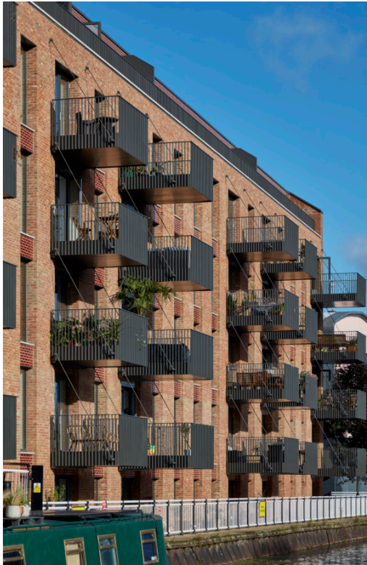
Bream Street, AHMM Ltd © Rob Parrish
