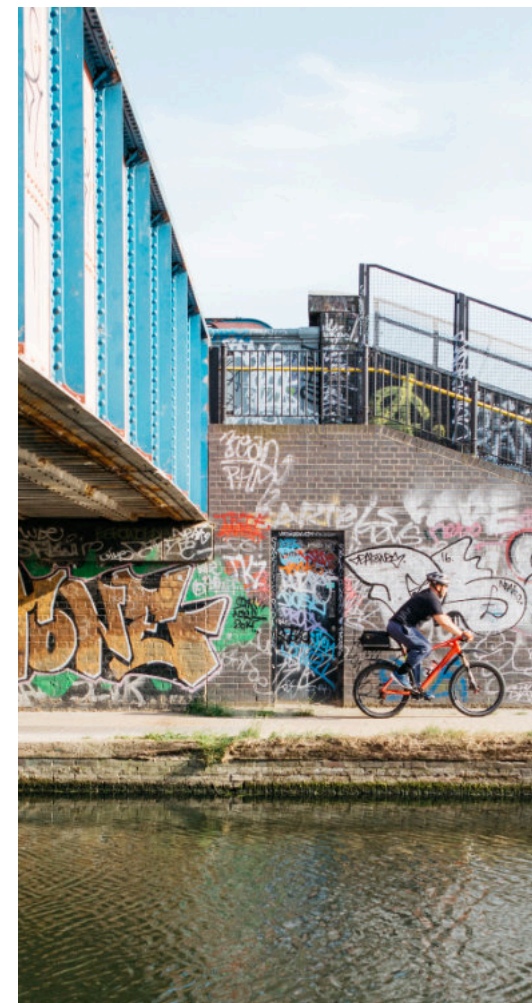
Mitre Bridge over the Grand Union Canal © Mattr Media Ltd
