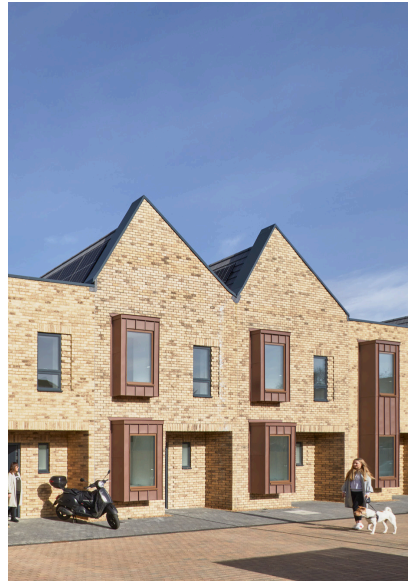
Underwood © Fuse Architects
