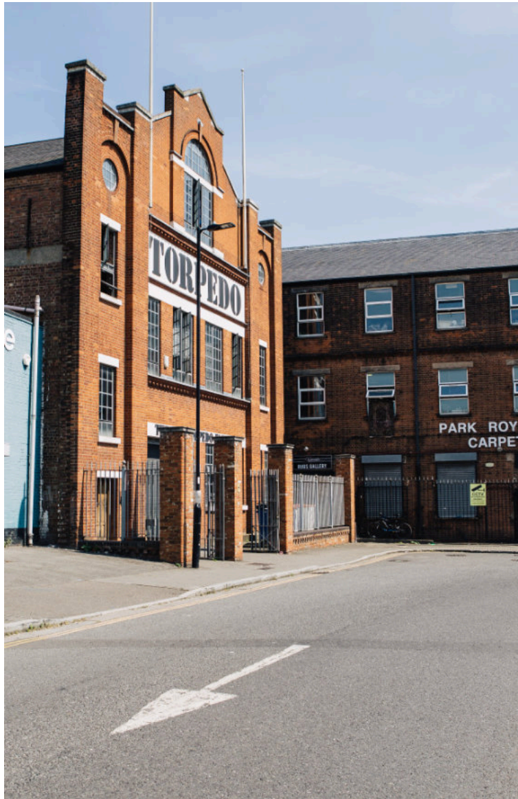
The old Torpedo Factory, a local heritage asset © OPDC by Mattr Media Ltd
