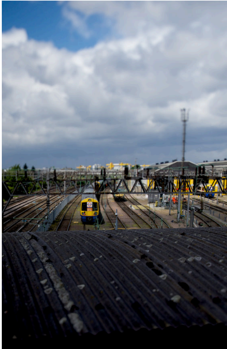
View of existing industrial and rail infrastructure at Old Oak © Mattr Media
