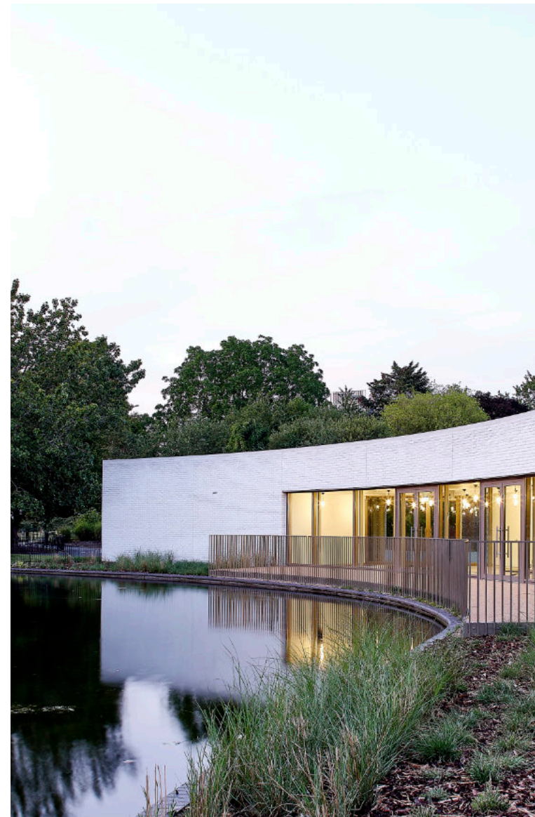
Southwark Park Pavilion, Bell Phillips Architects © Kilian O'Sullivan
