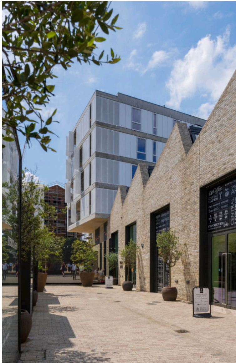
Rich Industrial Estate © London Square Developments Ltd
