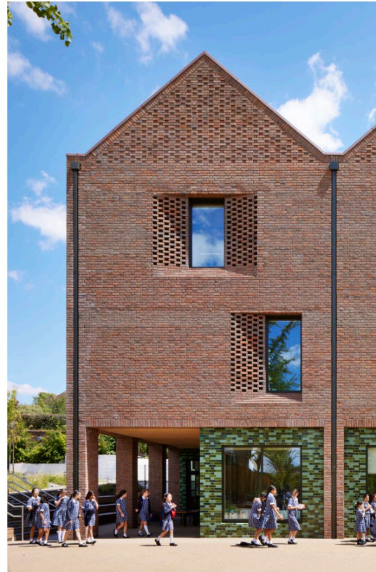
New Junior School for Notting Hill & Ealing High School, Hawkins\Brown © Jack Hobhouse
