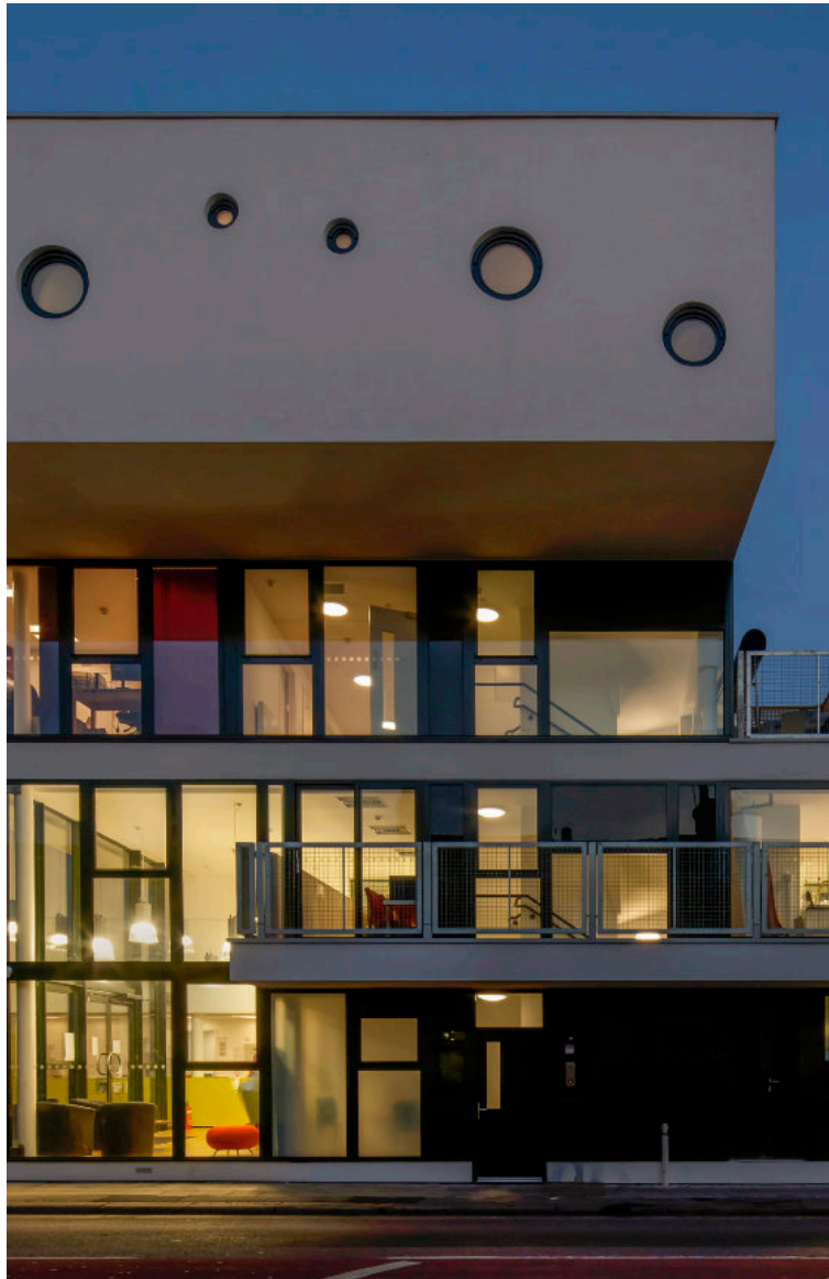
Redbridge Welcome Centre, Peter Barber Architects © Morley von Sternberg
